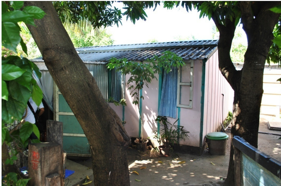
Photo 1 Cité La Mivoie - typical 1960s house made with asbestos panels
